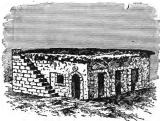
Dirt Covered House.
